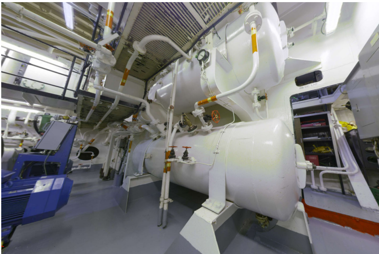
Figure 2 Existing Air Receivers
