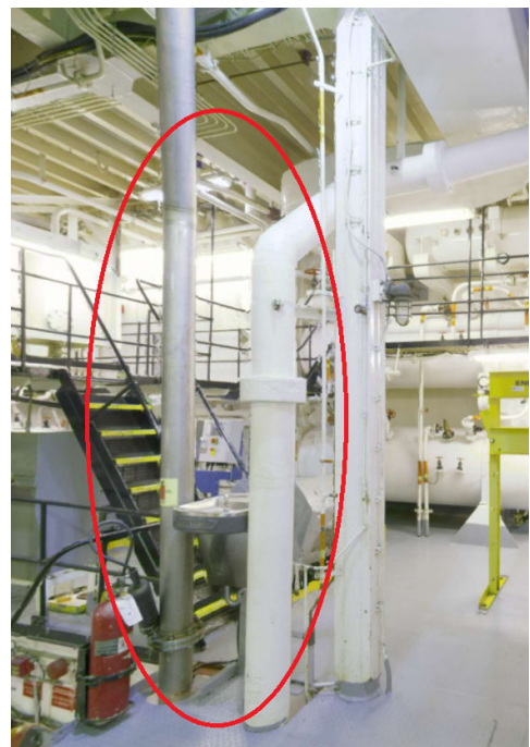
Figure 5 Vertical Pipes to be Removed
