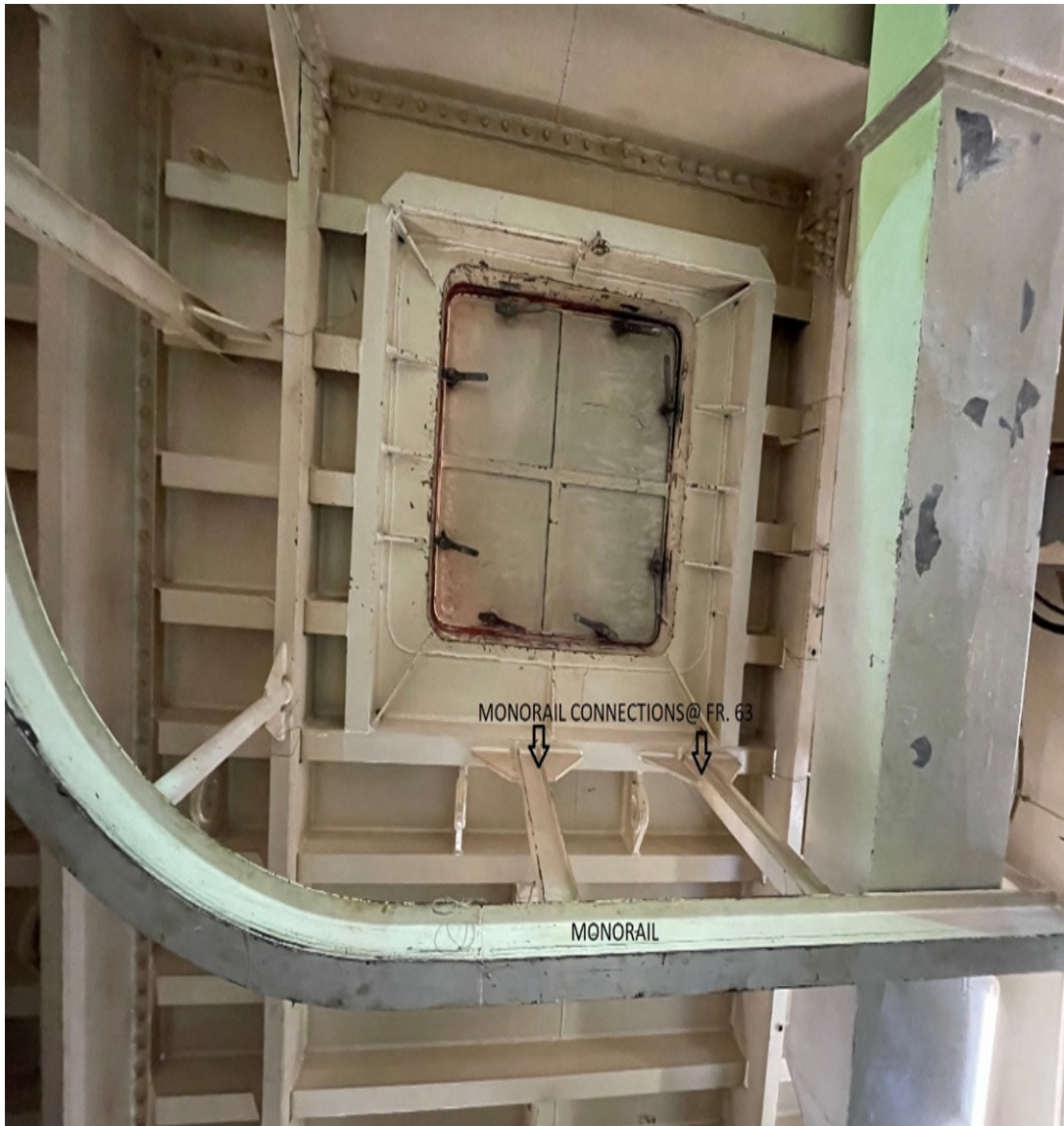
Picture 3.2.2 (Hatch underside)
