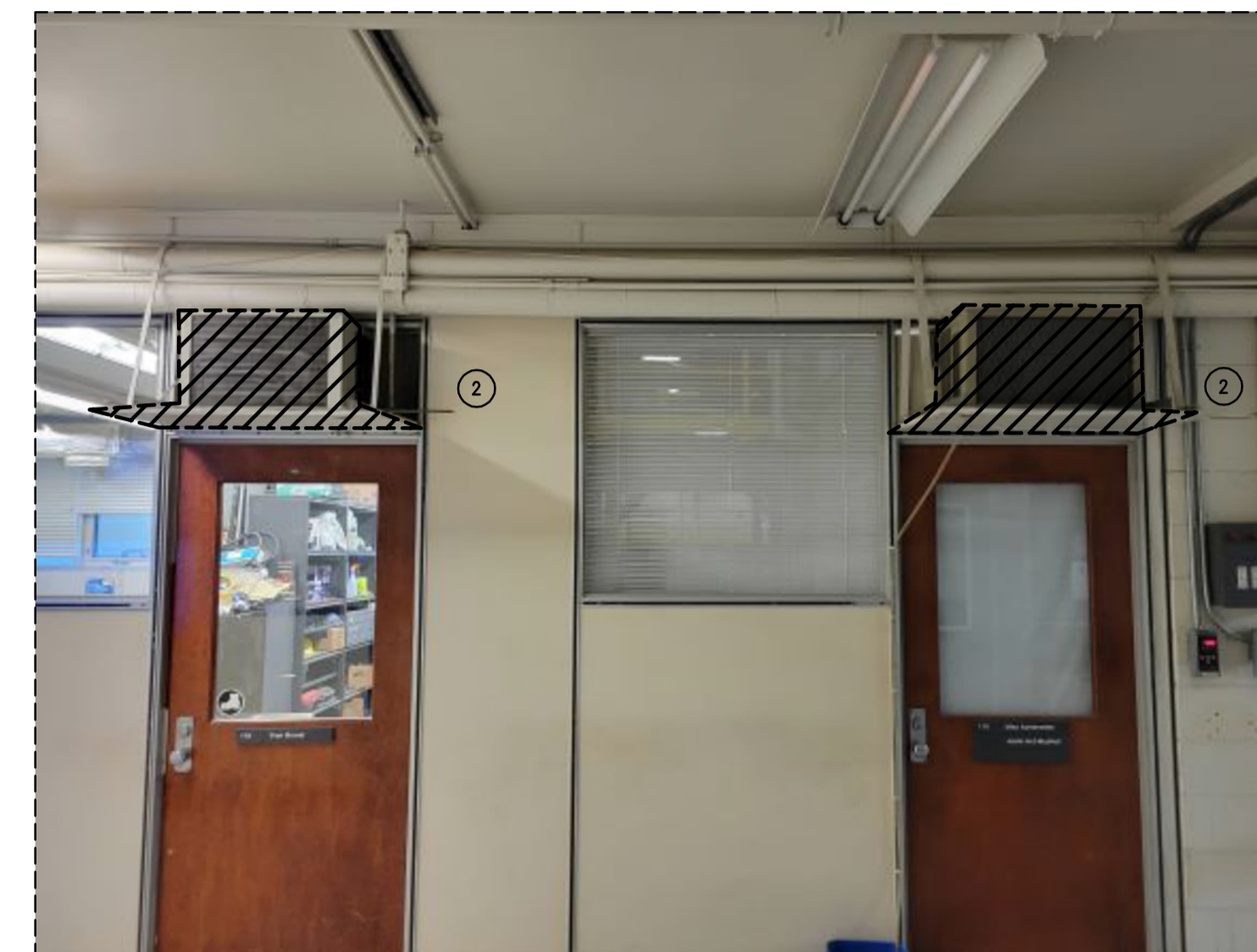
3 PHOTO NO. 2 - EXISTING WINDOW AIR CONDITIONERS REMOVAL M02 SCALE = N.T.S.
