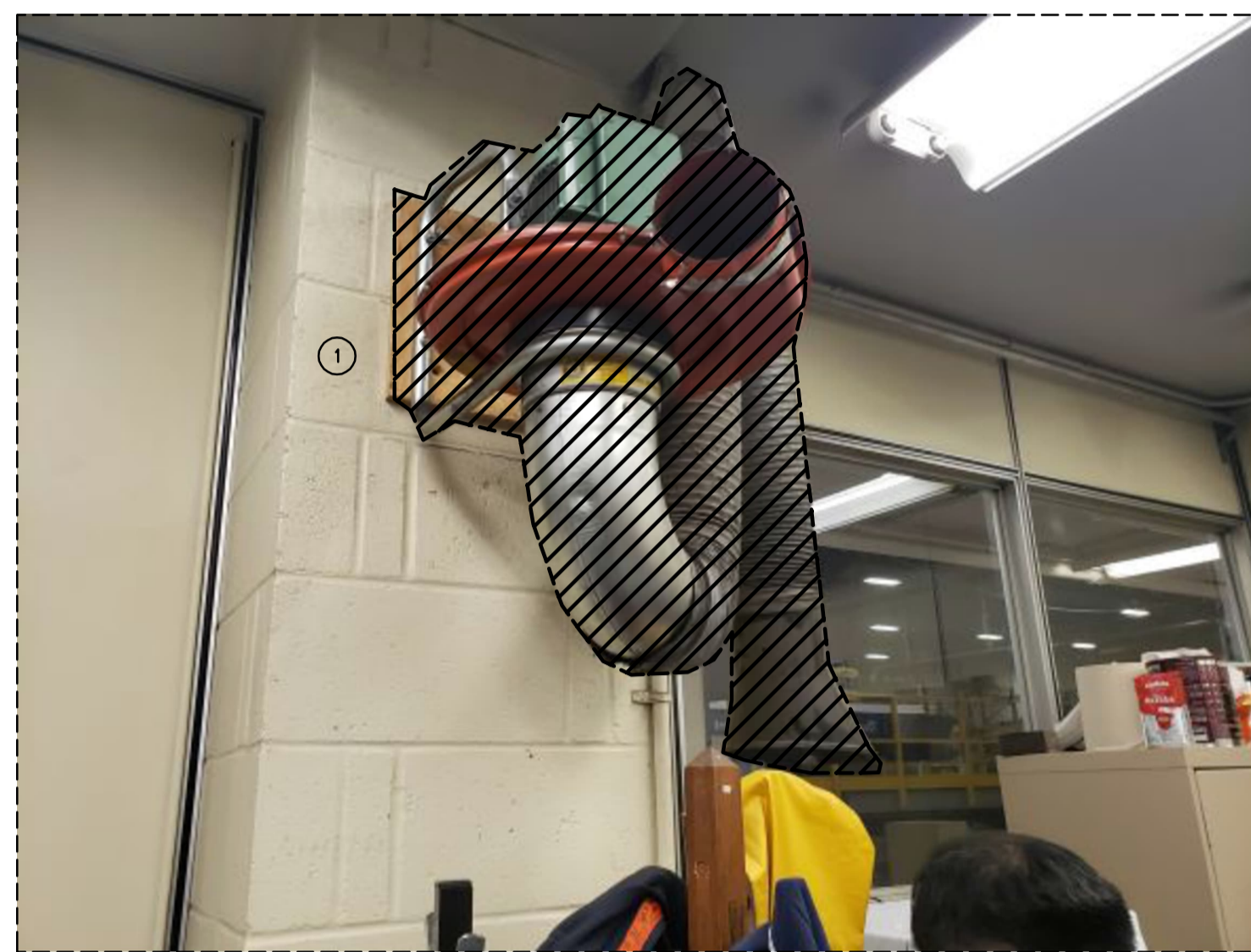
2 PHOTO NO. 1 - EXISTING EXHAUST FAN REMOVAL M02 SCALE = N.T.S.
