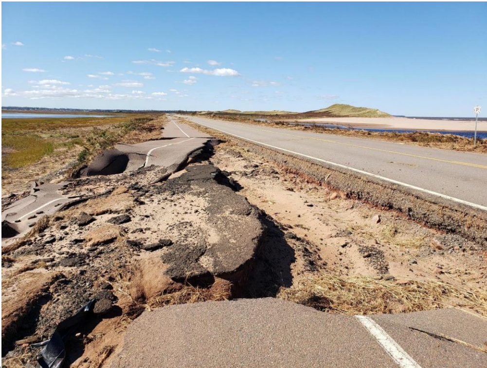
Figure 7. Storm damage to Multi-use trail on north side of Gulf Shore Parkway, west of Covehead bridge, post Hurricane Fiona. A) view looking east B) view looking west.
