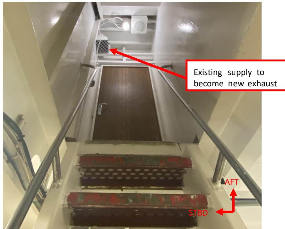
Figure 2: Sewage Compartment Entrance – View Looking Aft
