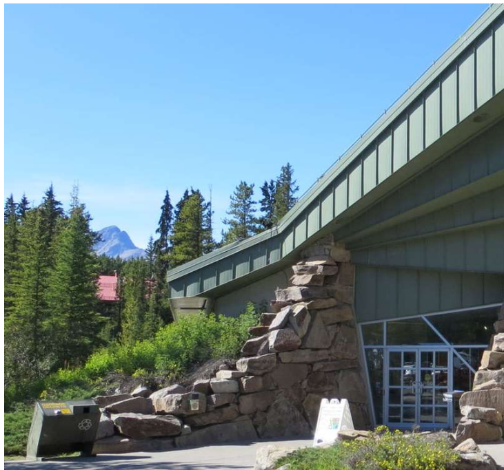
Figure 5. Image of installation location at Lake Louise Visitor Centre, located where garbage bins are. No AC power available, solar only.
