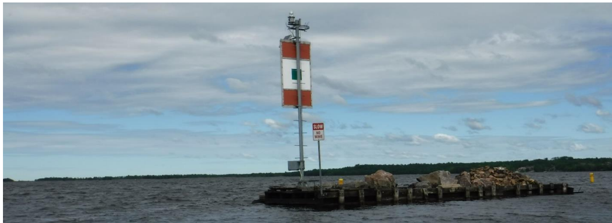
Figure 1: Existing AtoN Tower and damaged breakwater
