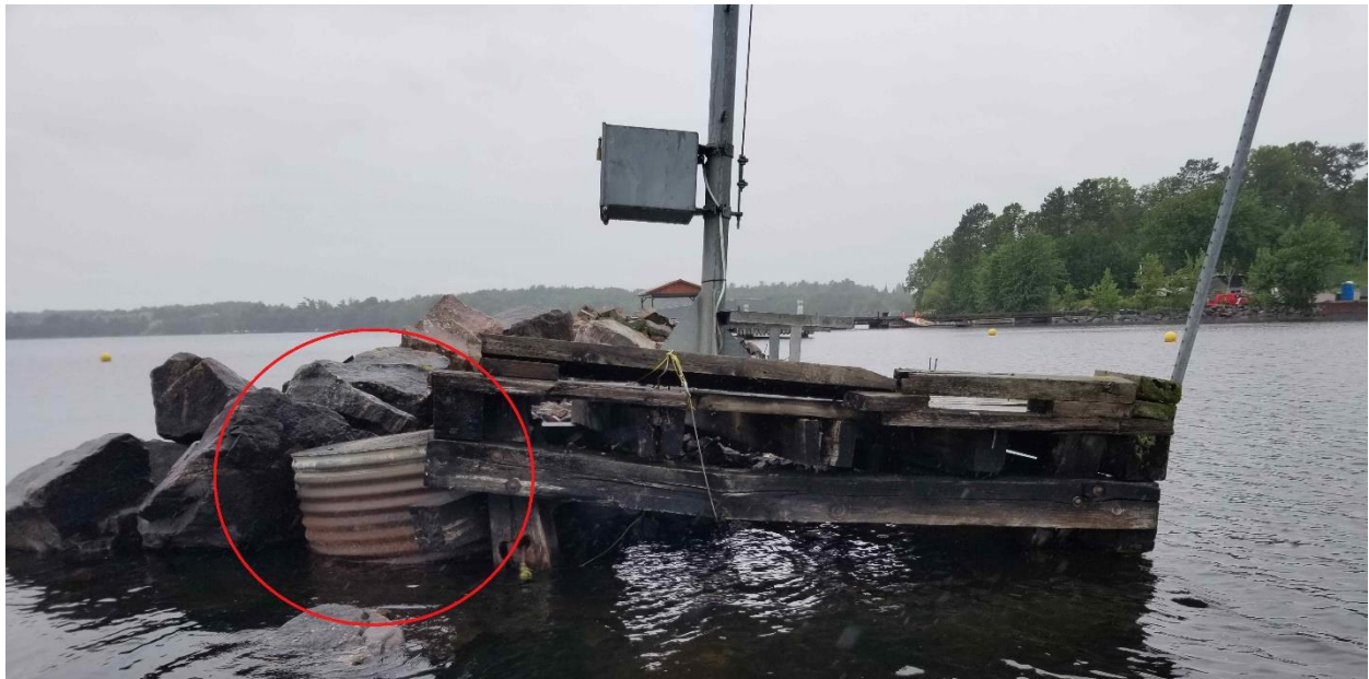
Figure 2: Existing wooden dock and abandoned concrete foundation.
