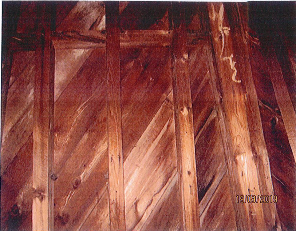
Photo 5: Alternate view of the 1 st floor walls and beams.
