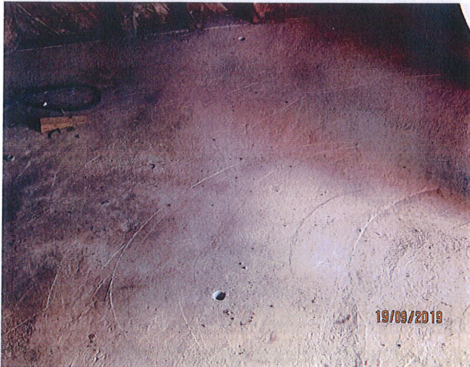
Photo 8: View of the concrete floor of the 1 st level.
