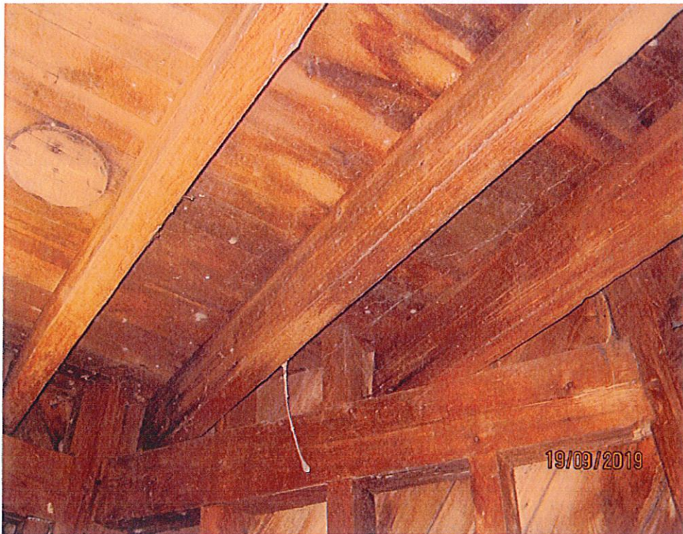
Photo 6: View of the ceiling of the 1 st level.
