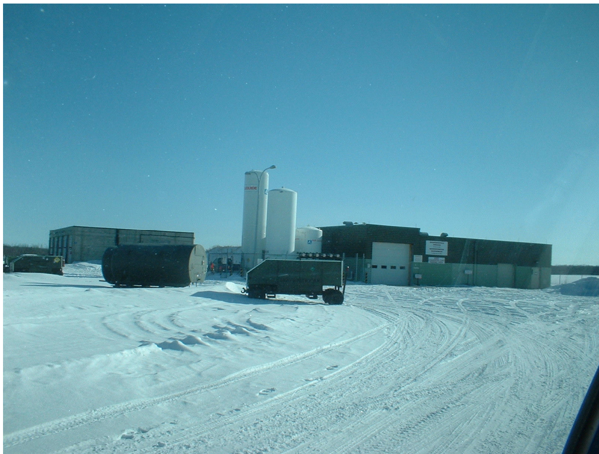
4th Wing Cold Lake, AB. LOX Facility.
