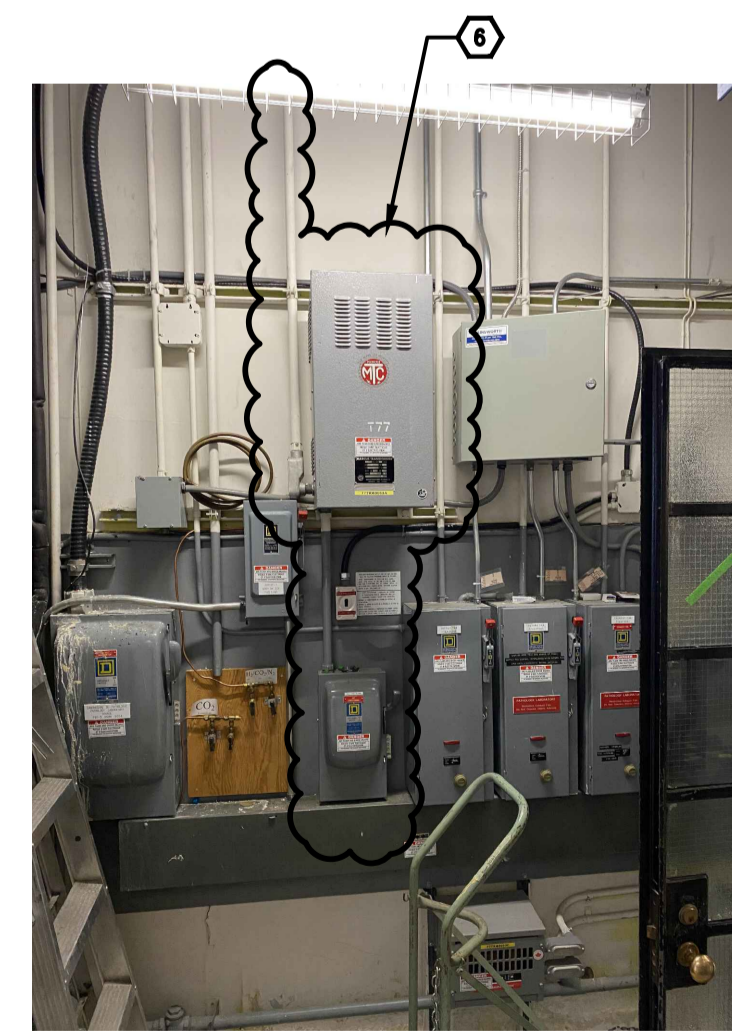
ROOM 3053 ELECTRICAL DEMOLITION WORK
