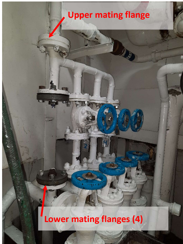
Figure 15.5.A – PW Manifold in ER
