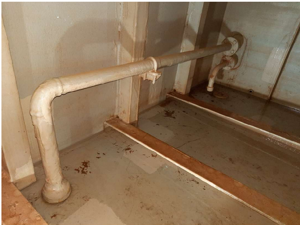
Figure 15.5.H – #1 PW line section and intake bell.
