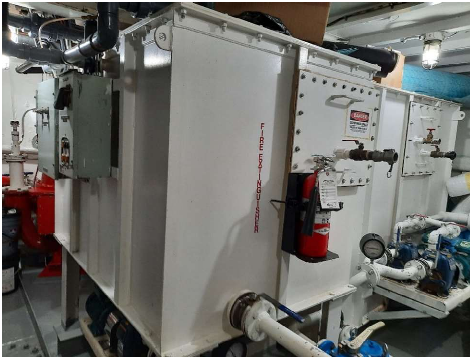
B1: Grey- & Black-Water Tanks overview, showing access doors
