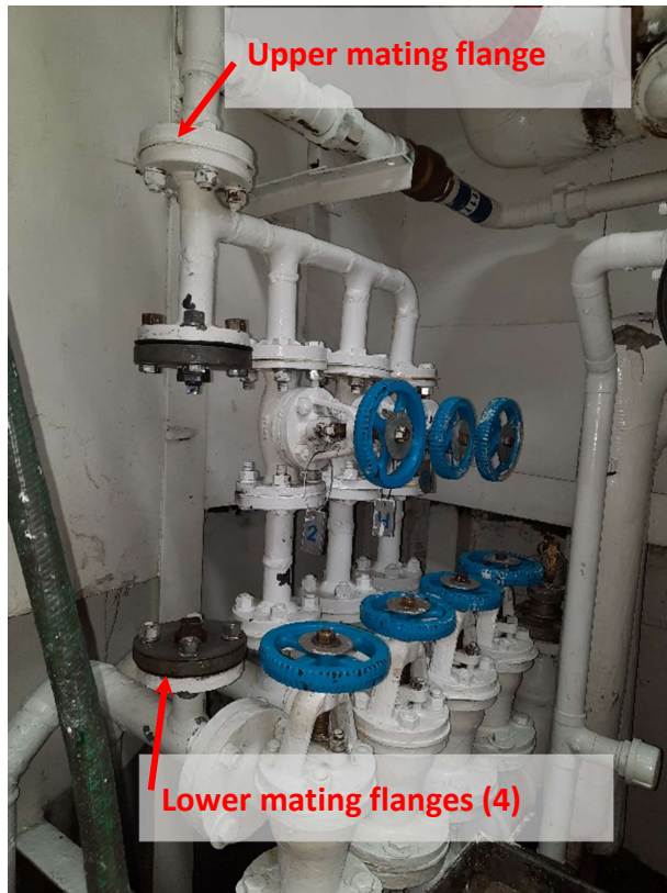
Figure 15.5.A – PW Manifold in ER
