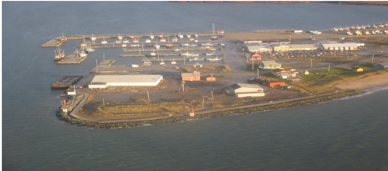
Figure 2.16 Photo of the West Sector of the Fishing Harbour - Point Area 2005
