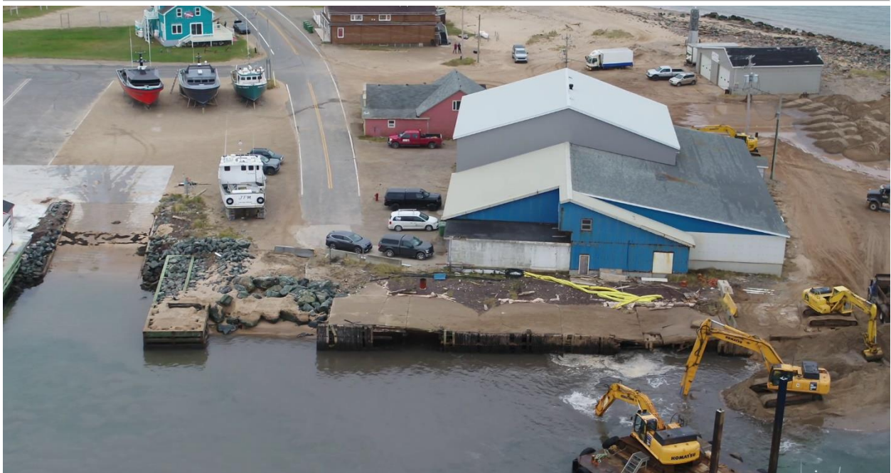
Figure 2.2 Photo of the West Sector of the Fishing Harbour - Ramp Area
