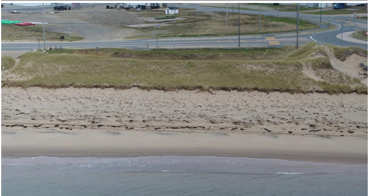
Figure 2.14 Photo of the western sector of the fishing harbour - Beach area
