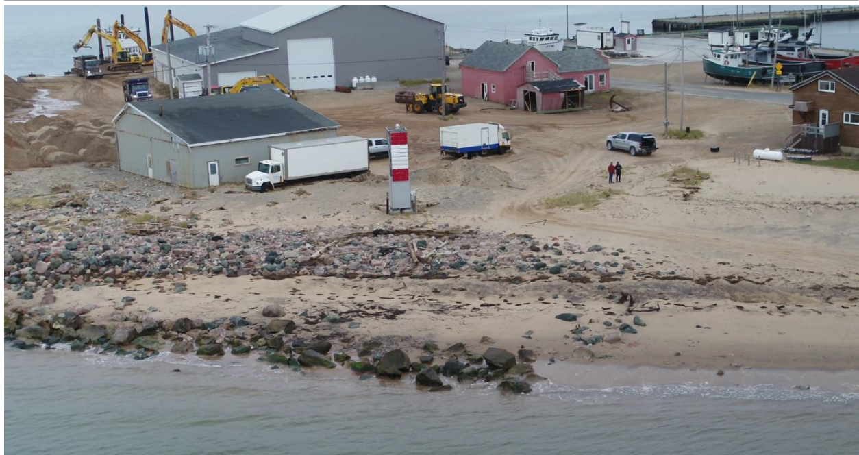
Figure 2.10 Photo of the West Sector of the Fishing Harbour - Rockfill Sector
