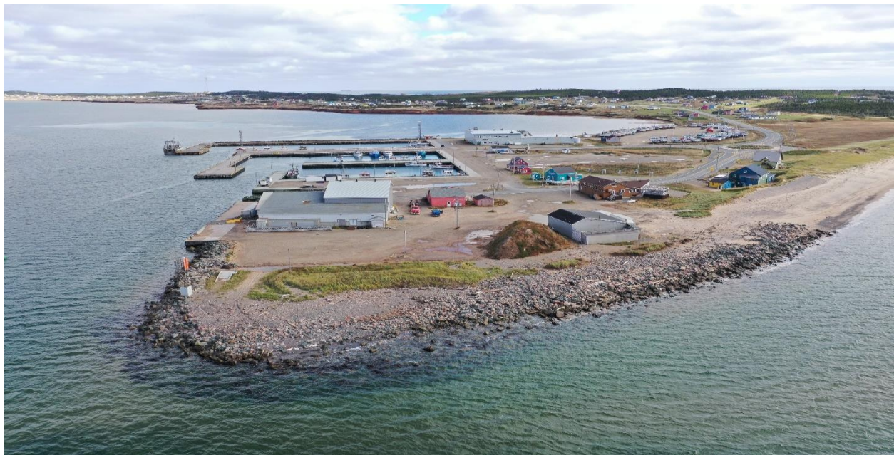
Figure 2.17 Photo of the western sector of the fishing harbour - Point sector in 2020 (Geoterram)
