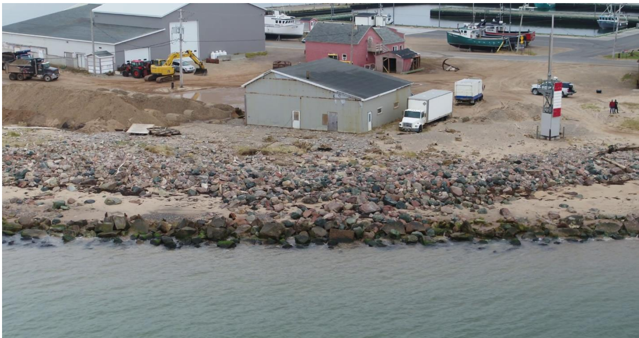
Figure 2.9 Photo of the West Sector of the Fishing Harbour - Rockfill Sector
