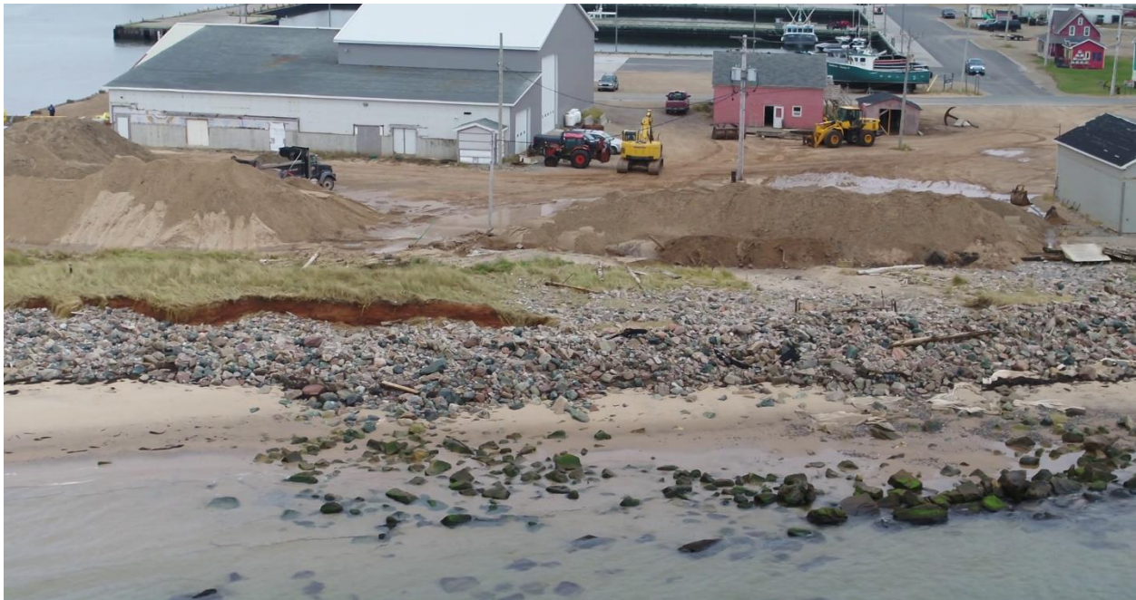
Figure 2.7 Photo of the West Sector of the Fishing Harbour - Rockfill Sector
