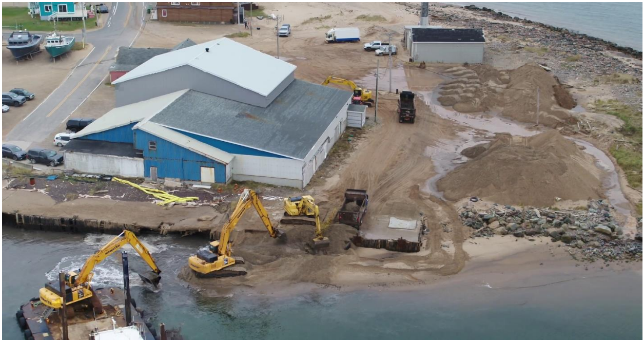
Figure 2.3 Photo of the west sector of the fishing harbour - Wharf area
