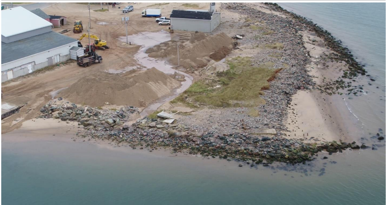
Figure 2.4 Photo of the western sector of the fishing harbour - Pedestrian area
