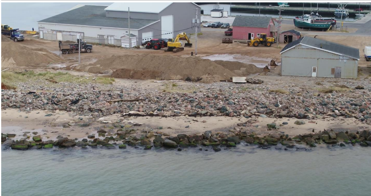
Figure 2.8 Photo of the West Sector of the Fishing Harbour - Riprap Sector
