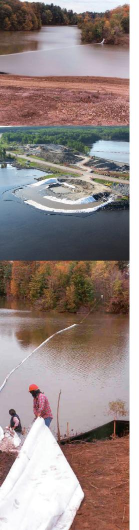
**terrafix**® Silt Curtains are designed to deflect and contain sediment within a designated area. Manufactured from high strength geotextiles and fabricated to a variety of sizes.
