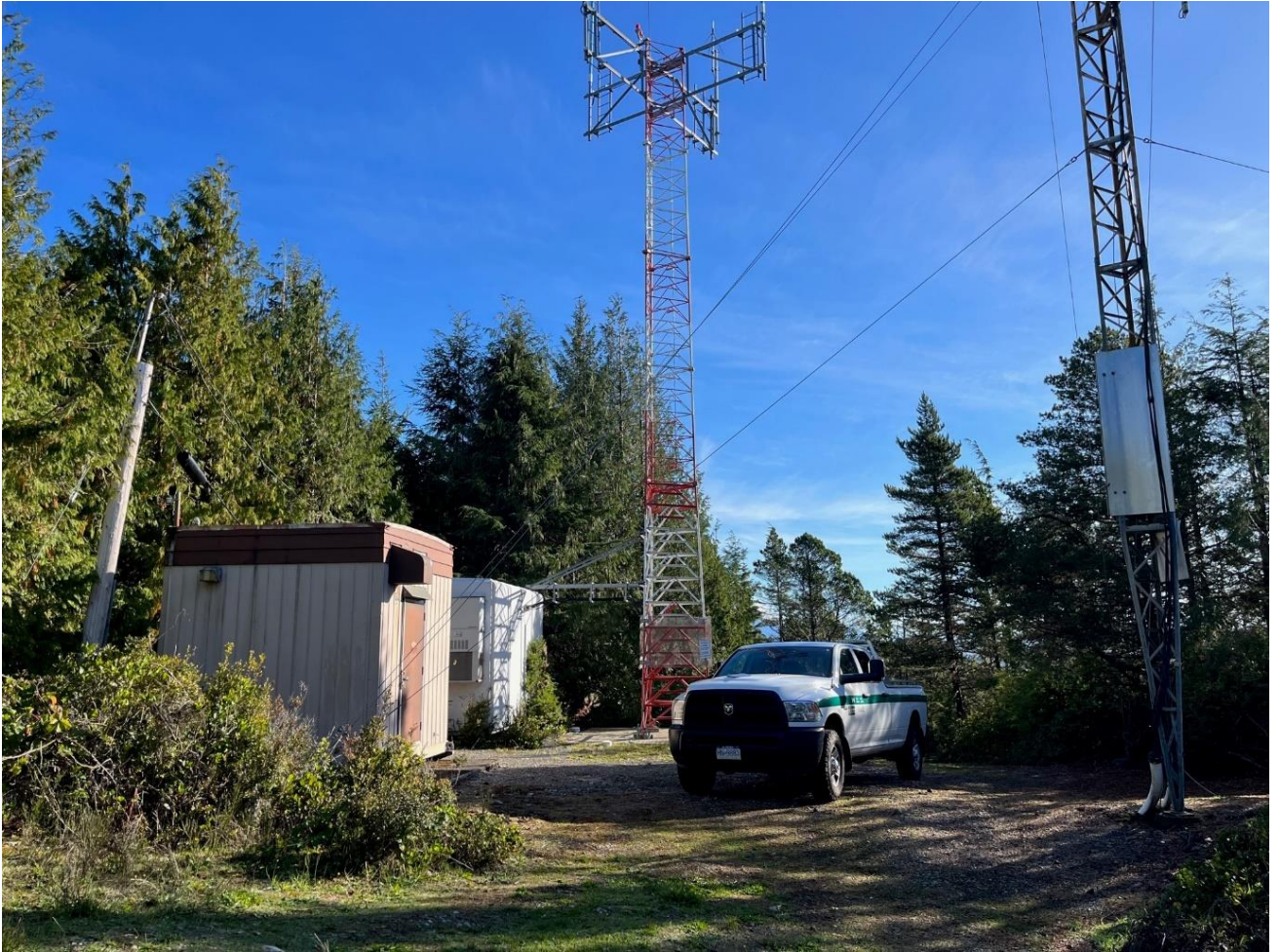
Figure 3: View of Telegraph Hill site looking towards the access road. The NAV CANADA tower and shelter are shown in the background. The Telus tower and shelter in the foreground will be decommissioned and removed from the site prior to January 1 st , 2024.
