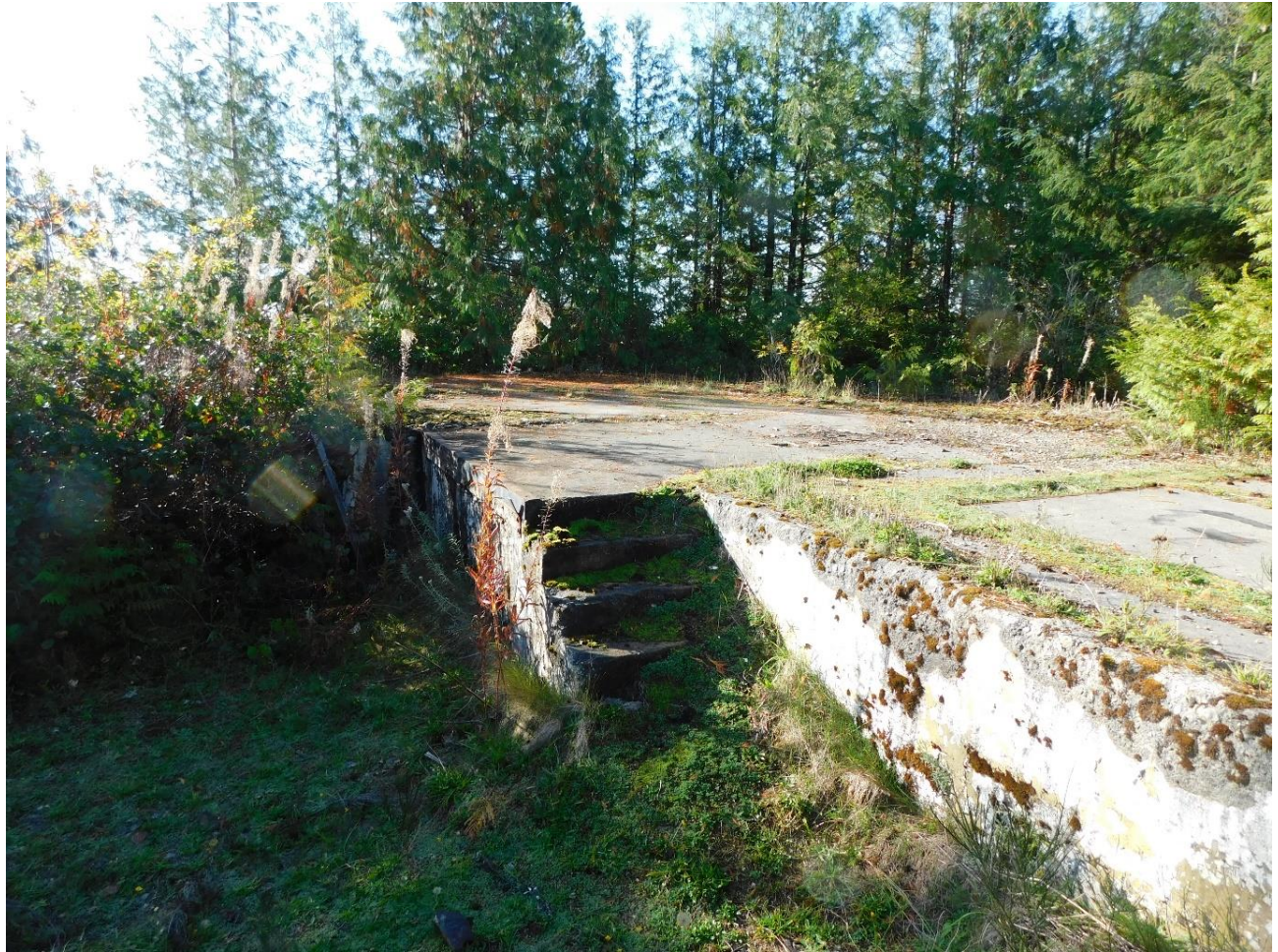
Figure 6: Side view of concrete pad.
