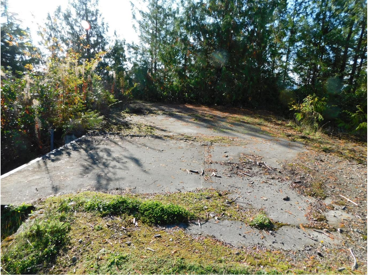
Figure 5: Top view of concrete pad.
