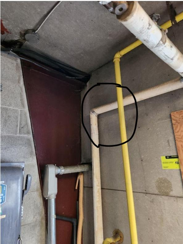
Cement paste of the heating pipe that will be removed by AAFC
