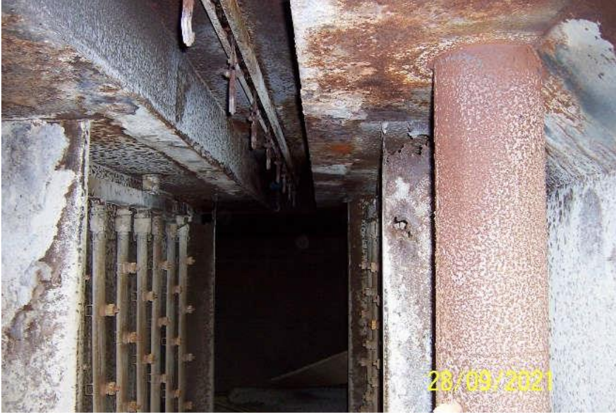
Photo 1 - Interior of Unit 1 (Stage #1) Upper part
