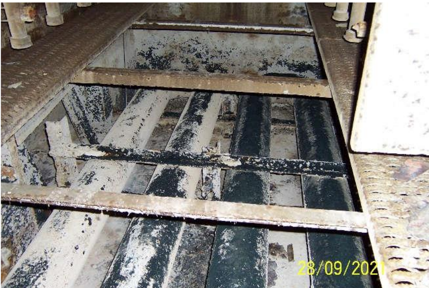
Photo 2 - Interior of Unit 1 (Stage #1) Lower part
