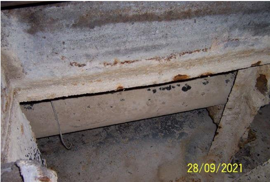
Photo 3 - Basin of Unit 1 (Stage #1)
