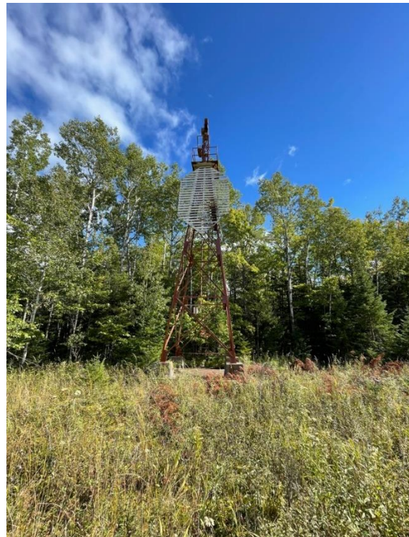
Figure 4: Existing LL5417 Rear Range Tower
