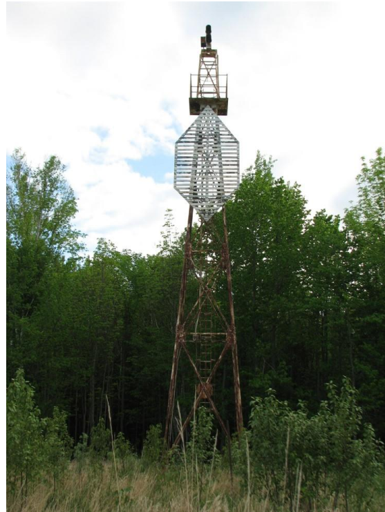
Figure 2: Existing LL5415 Rear Range Tower
