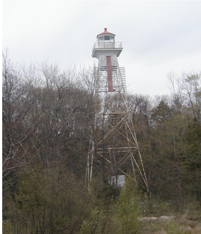
Figure 3: Tower site looking from straight on.
