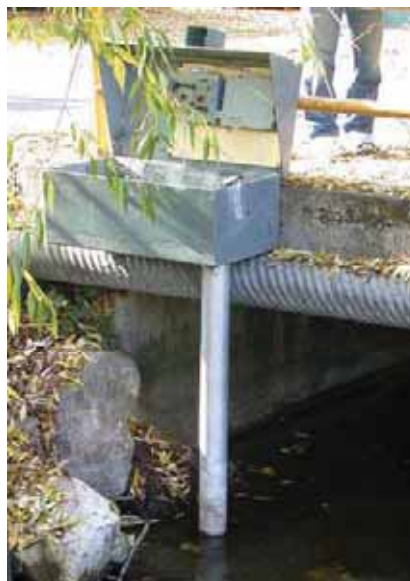
Figure C-3. A sturdy box that contains an external data logger and battery can be used to protect the equipment. Photo: Linda Gregory
