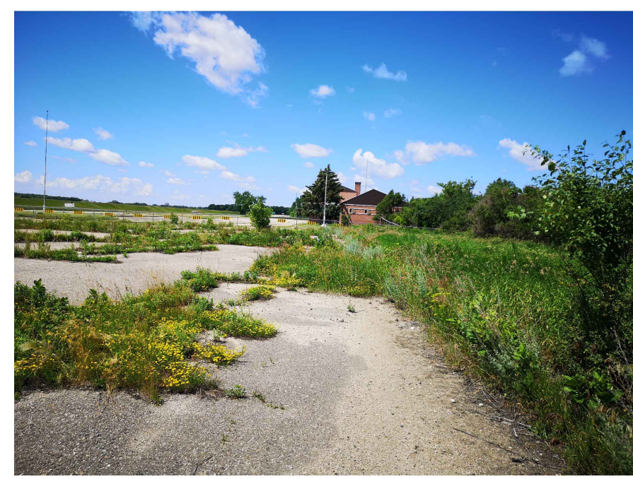
1 TYPICAL VEGETATION ON CONCRETE PAD
