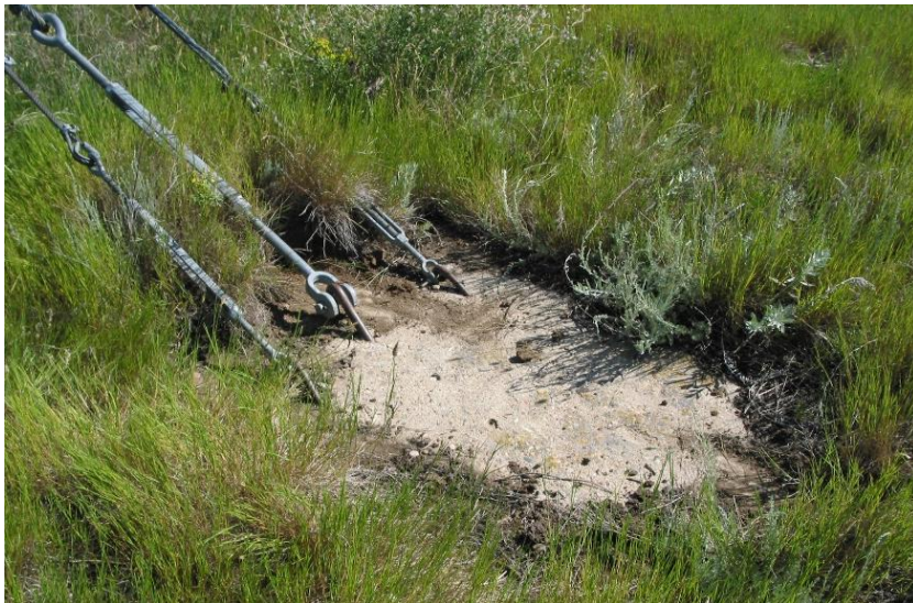
Figure 8. Post attached to concrete pad on right bank far side
