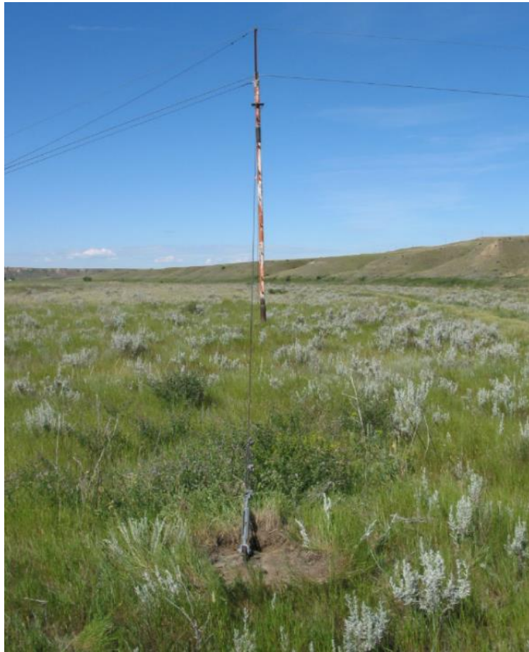
Figure 7. Main Center Concrete anchor on right bank far side
