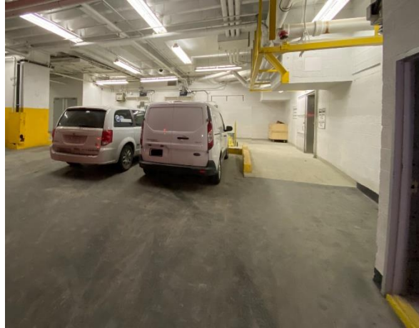
Photo 2 : Photo taken from the loading dock door with a view of the inside of the loading dock area
