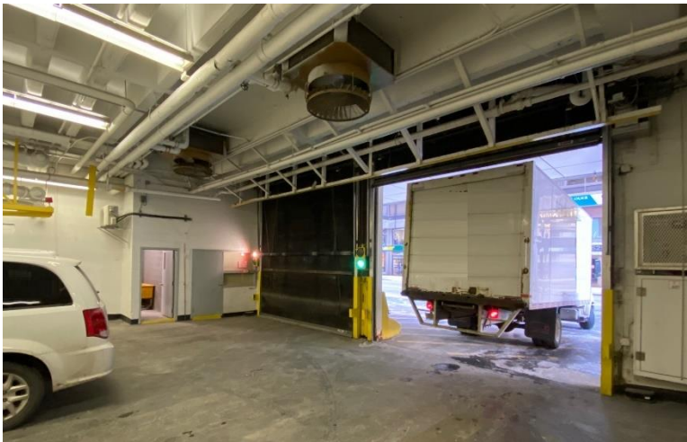
Photo 3 : Photo of the loading dock door taken from the inside
